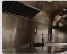
Stainless steel wall
